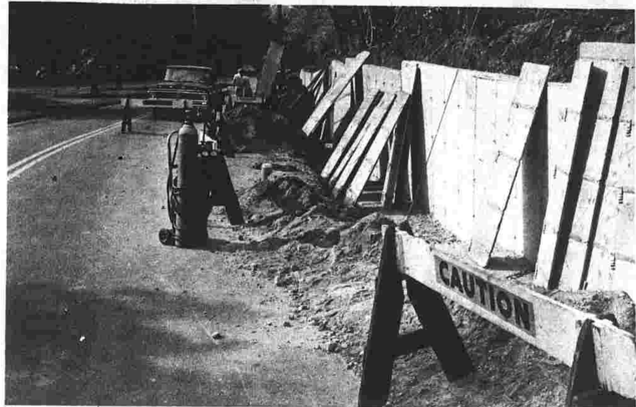
Retaining wall under construction
